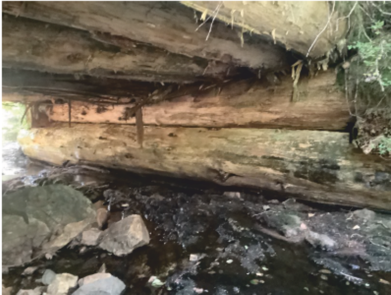
Right Bank Abutment when facing downstream
