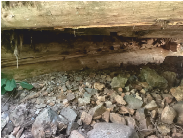
Left Bank Abutment when facing downstream
